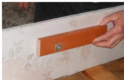
Drilling and fixing through an additional backing plate adds strength behind an MDF side
