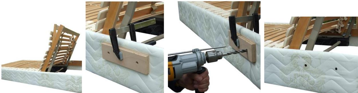
*Raise action out of the way – clamp template – drill through template – nice clean holes for bolts!*
